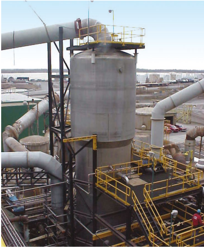
ZeCor® towers and pump tanks can be shop fabricated prior to plant shutdown and staged on-site for insertion of Brink® mist eliminators, UniFlo® acid distributors and tower packing.
